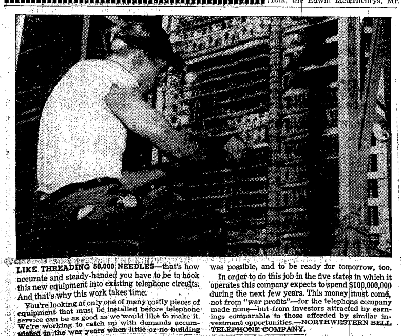
LIKE THREADING 50,000 NEEDLES—that's how accurate and steady-handed you have to be to hook this new equipment into existing telephone circuits. And that's why this work takes time. You're looking at only one of many costly pieces of equipment that must be installed before telephone service can be as good as we would like to make it. We're working to catch up with demands accumulated in the war years when little or no building was possible, and to be ready for tomorrow, too. In order to do this job in the five states in which it operates this company expects to spend $100,000,000 during the next few years. This money must come, not from "war profits"—for the telephone company made none—but from investors attracted by earnings comparable to those offered by similar investment opportunities.—NORTHWESTERN BELL TELEPHONE COMPANY.
